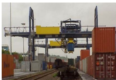
Picture 2: Crane systems
